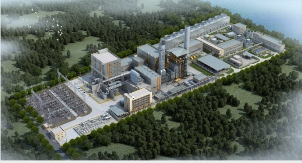
Architectural rendition of Summit Meghnaghat II Power Co Ltd (583MW) to be powered GE's 9HA gas turbine.
